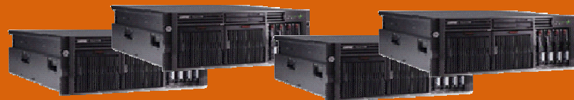
CRM application server farm
